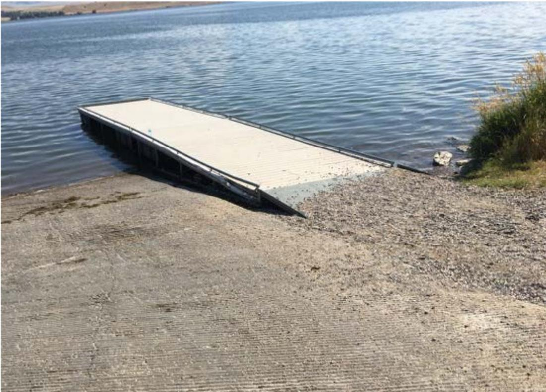
Most of the remaining damage is underneath the dock but you can see the damaged rail and side bumper.
